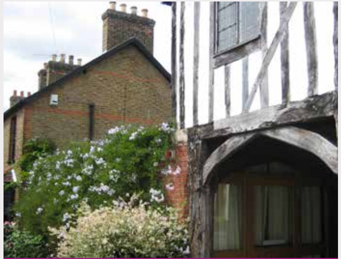
A rich palette of materials and historic building types, Horndon on the Hill
