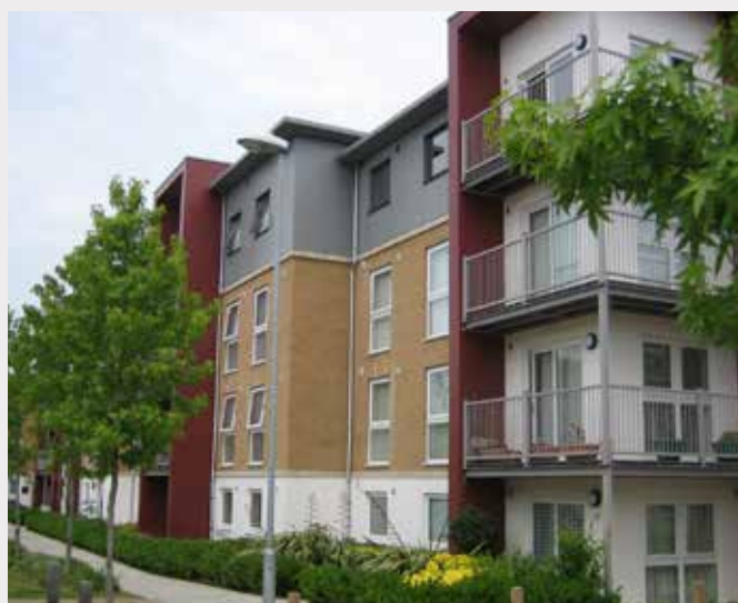
Defined corner at junction of streets, Grays
