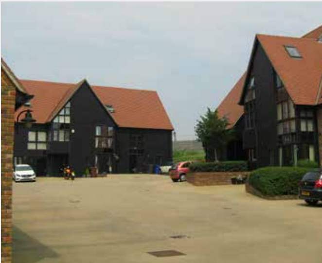
An acoustic fence has been carefully integrated for HS1
